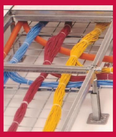
FloorFlex is the product of years of fine tuning and hands on experience in the access flooring industry. In the past, overhead tray systems had to be modified for use in traditional access floor systems, resulting in high material cost, increased labor time and poor system integration. FloorFlex is innovative in it's usage of highly engineered simple to install components that makes our cable tray systems the most effective installation and maintenance solution.
